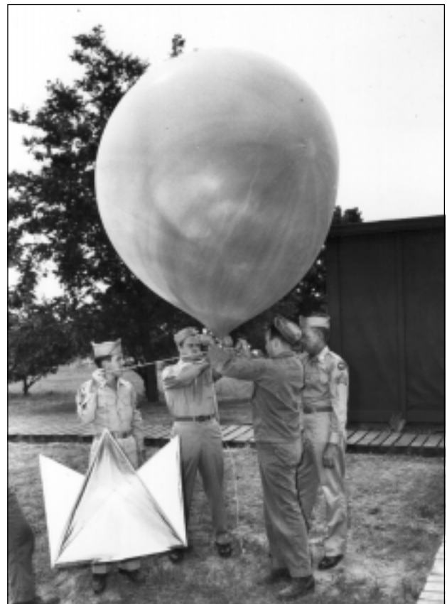
Figure 1. A neoprene weather balloon and a 1947-era rawin radar target.
